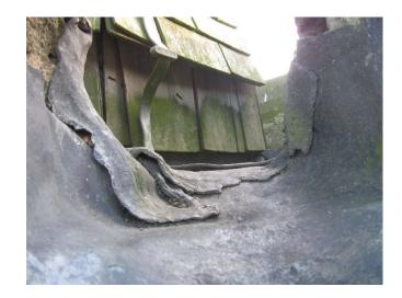
As the picture shows, the wooden base of the Spire needs to be replaced. In addition, the shingles are old, and some are split, they need replacing on new boarding to make them watertight.
